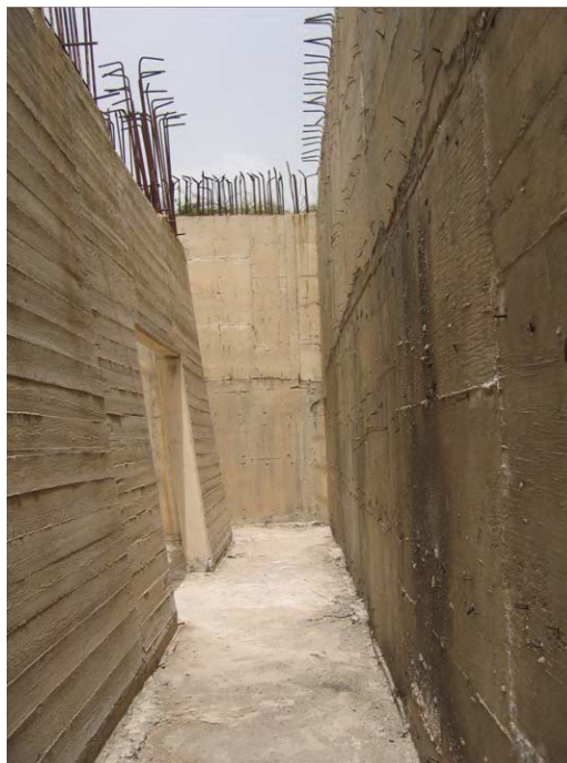
Figure 2. Pasargadae Archaeological site museum, sloping wall of unfinished building. Photograph by authors 2004.
